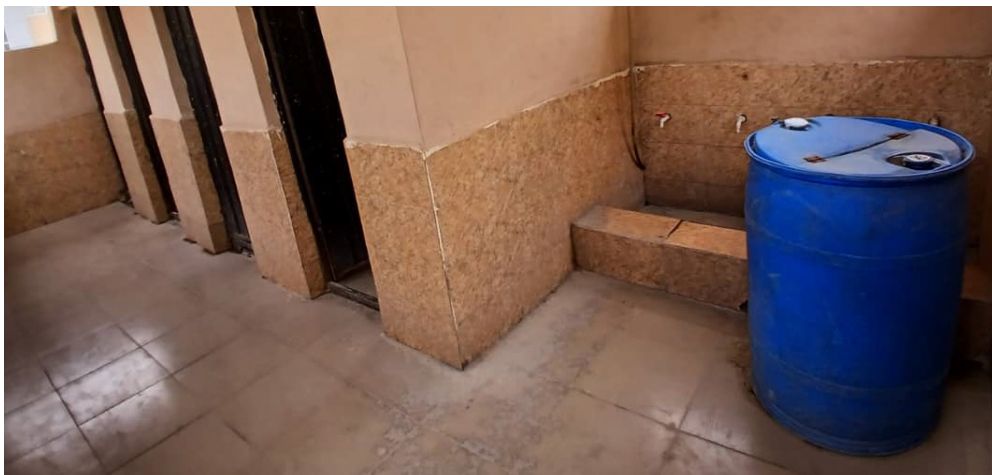
High Court Toilets
