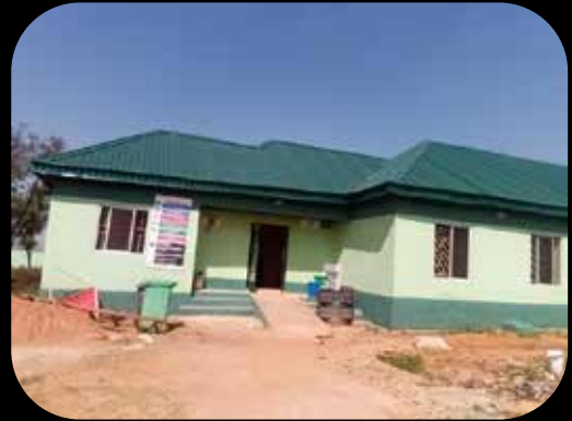
Renovated Gidan Tagwai PHC (Front View)
