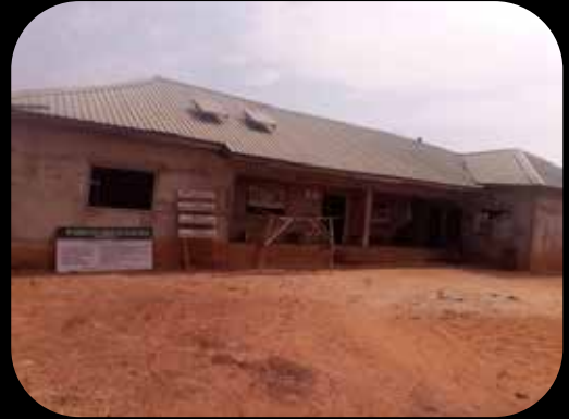
Previous Gidan Tagwai PHC (Front View)
