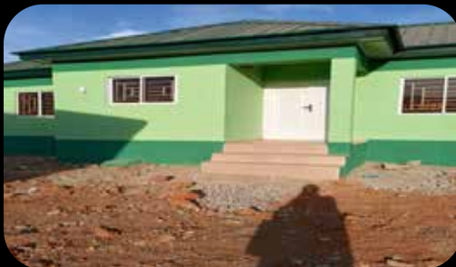
Renovated Sabon Tasha Primary Health Care Centre
