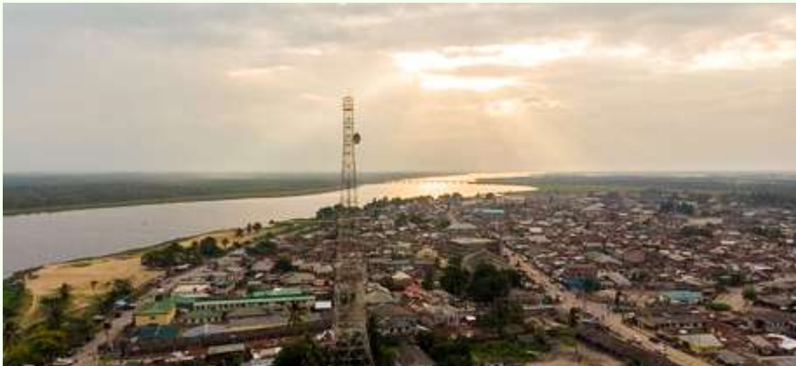
Figure 1: An aerial view of Badagry, Lagos State (Source: pmnewsnigeria.com)
