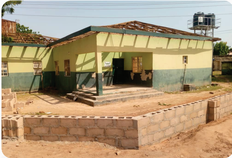
Ongoing Renovation of Gombe Abba PHC Facility
