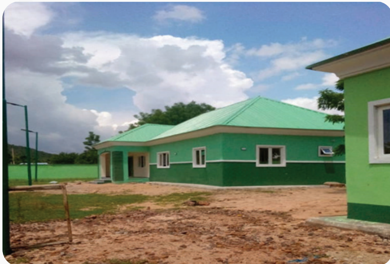
Construction of Staff Quarters at Gombe Abba PHCC.
