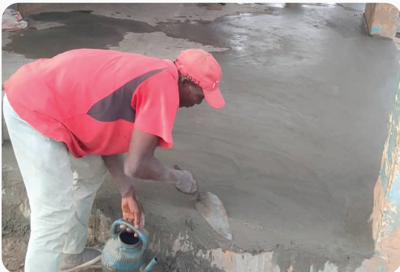
Ongoing renovation of the broken floor at PHC Kodo
