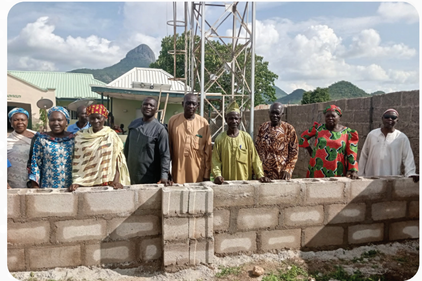
Ongoing facility fencing at Lapan PHC by Community Members.
