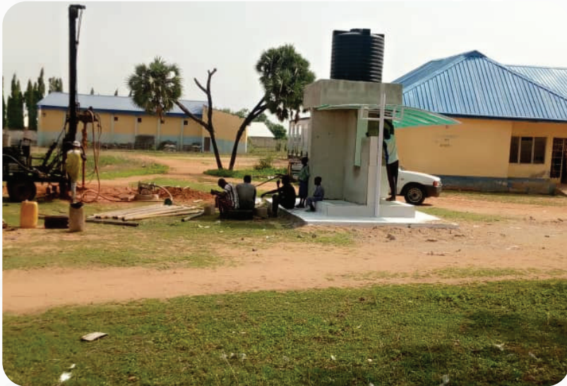
Provision of water borehole at MCH Sabon gari Wushishi LGA
