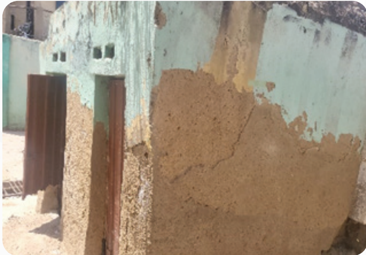
- Toilet Construction at Gwagwarwa PHC
