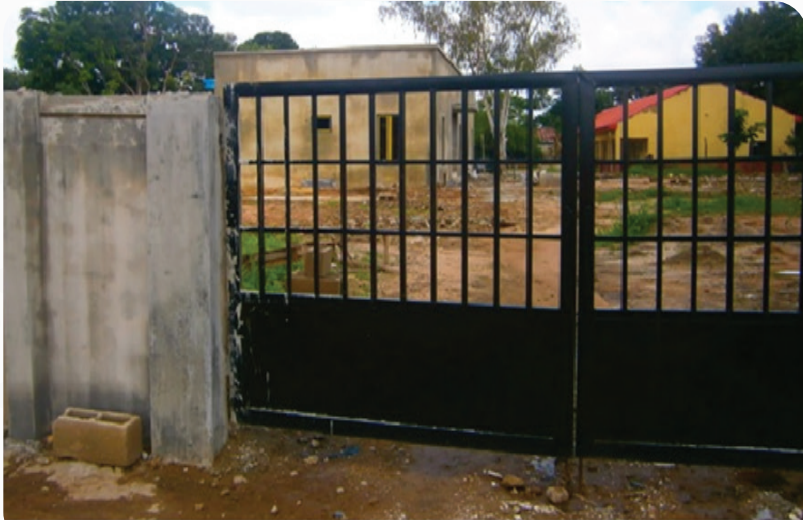
Reconstructed School MCH Limawa A, for commissioning soon Aug '24
