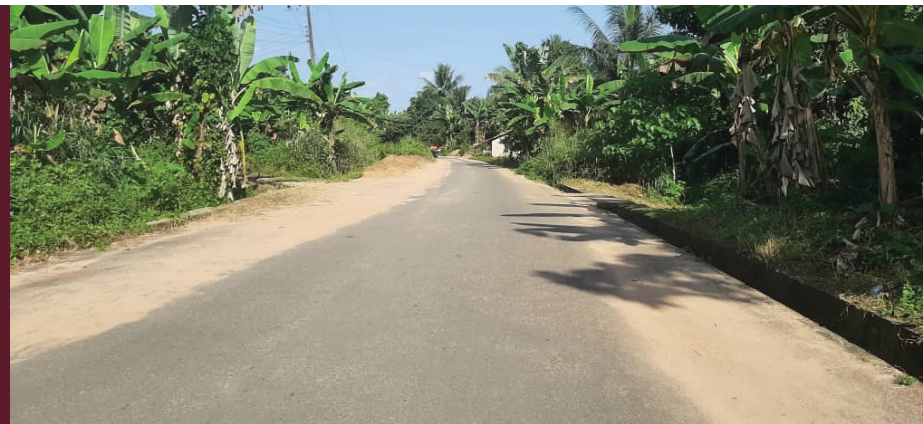
The road after completion with good drainages
