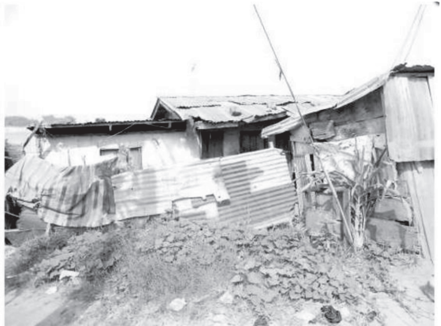
Affected building in Atani Community
