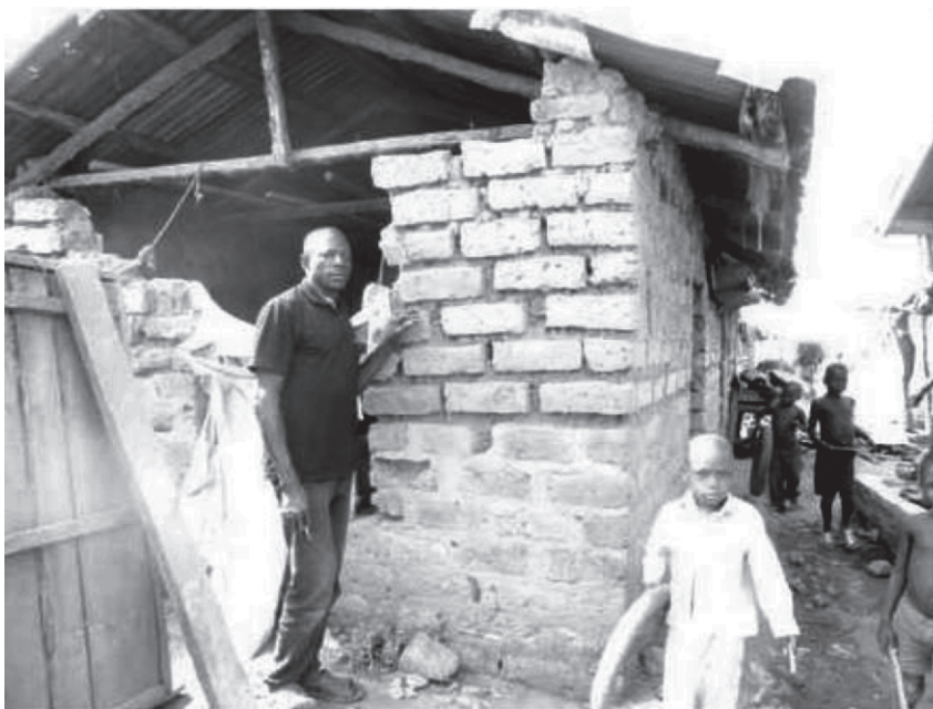
Affected building in Ijiwo Vilage, Akpe LGA
