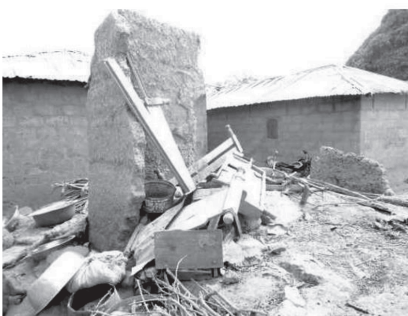
Affected Building in Ketso Area, Mokwa LGA
