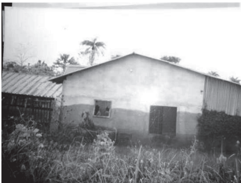
A Flooded House in Ojene-Ibaji Village in Ibaji LGA
