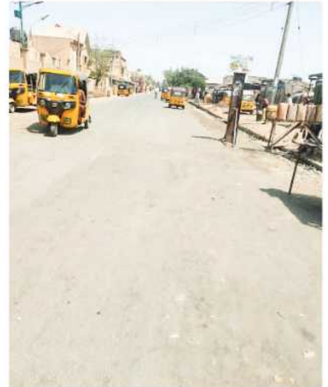
Less than 1Km Dan Fulani road at Tarauni LGA (Amount: N50m)
