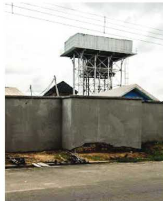
The completed Abonema water project in Rivers State (Amount: N90m)
