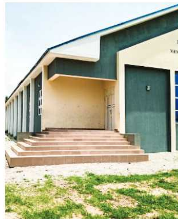
Newly constructed Mararaba Townhall, Donga LGA, Taraba State, named after Senator Emmanuel Bwacha (Amount: N100m)
