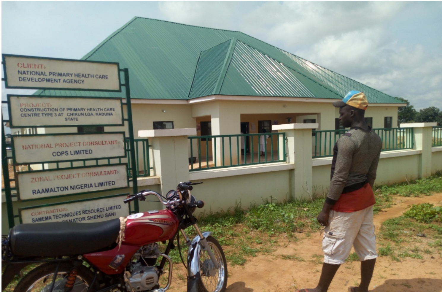
CONSTRUCTION OF PRIMARY HEALTH CARE CENTERS IN KADUNA CENTRAL SENATORIAL DISTRICT, KADUNA STATE
