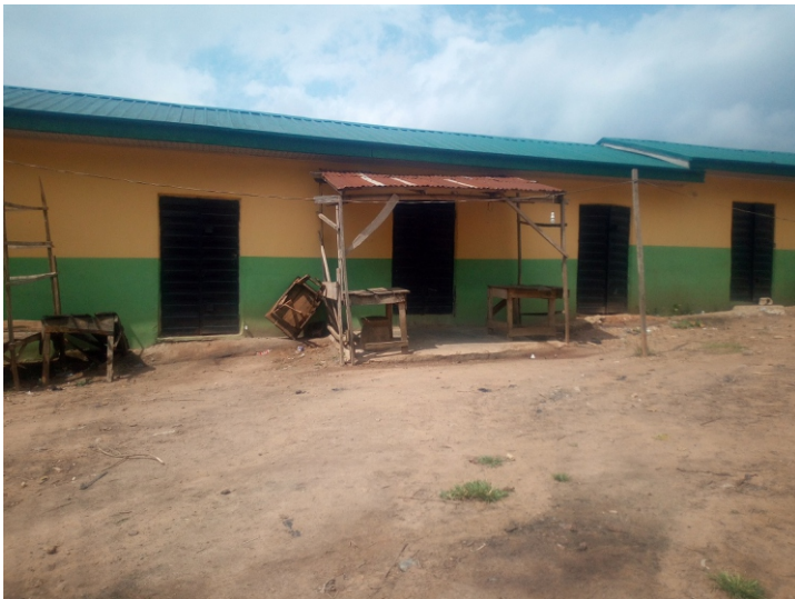
CONSTRUCTION OF LOCK UP SHOPS IN IKUNRIN EKITI IKOLEOYE FEDERAL CONSTITUENCY EKITI STATE
