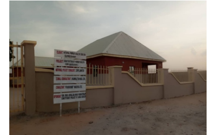
CONSTRUCTION OF TWO HOSTEL AT FEDERAL UNIVERSITY BIRNIN KEBBI.
