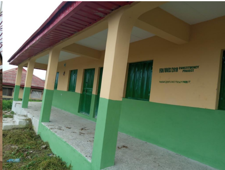
IPARA REMO COMPLETED CLASSROOMS
