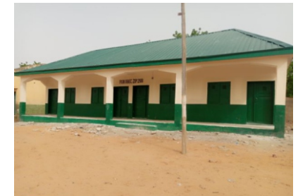
CONSTRUCTION OF TWO (2) BLOCK OF CLASSROOMS IN AUGIE LGA, KEBBI NORTH SENATORIAL DISTRICT, OF KEBBI STATE
