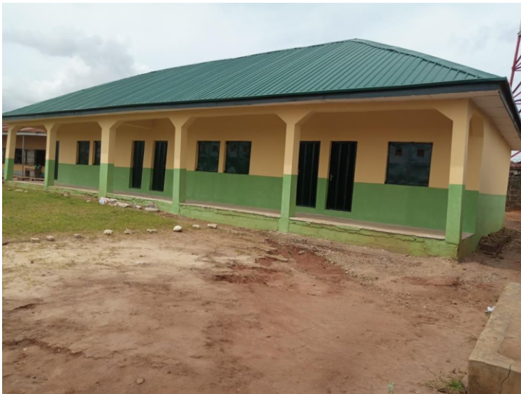
SAGAMU COMPLETE CLASSROOMS STRUCTURE
