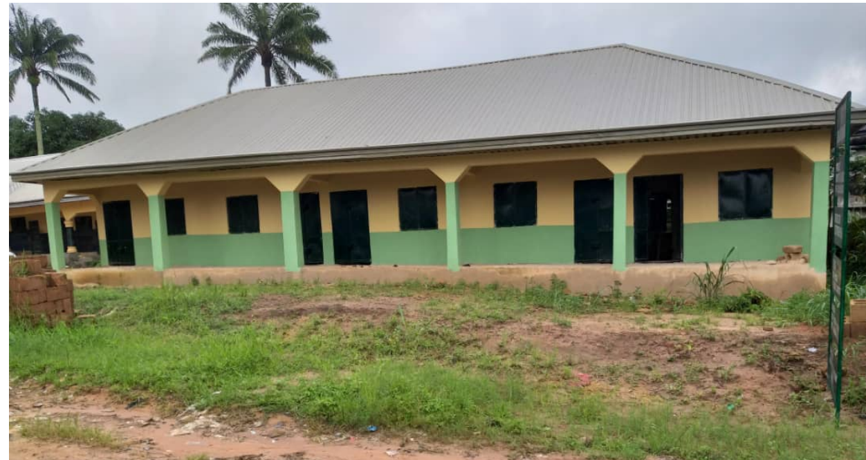
CONSTRUCTION OF FOUR(4) CLASSROOM BLOCK WITH HEADMASTER'S OFFICE IN UMUOHI-OKIJA, IHIALA FEDERAL CONSTITUENCY,ANAMBRA STATE.
