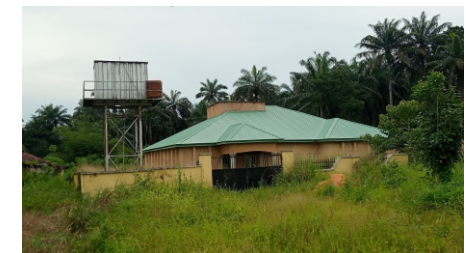
COMPLETION OF HEALTHCARE CENTRE AT UGIRI-IKE, IKEDURU LGA, IMO STATE (2)
