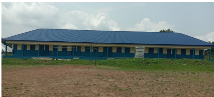
RENOVATION OF 2 CLASS ROOM BLOCK AT ST JOHN PRIMARY SCHOOL AKAMKPA
