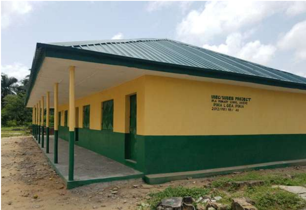
Renovated school in Ogun State in Akere Community.
