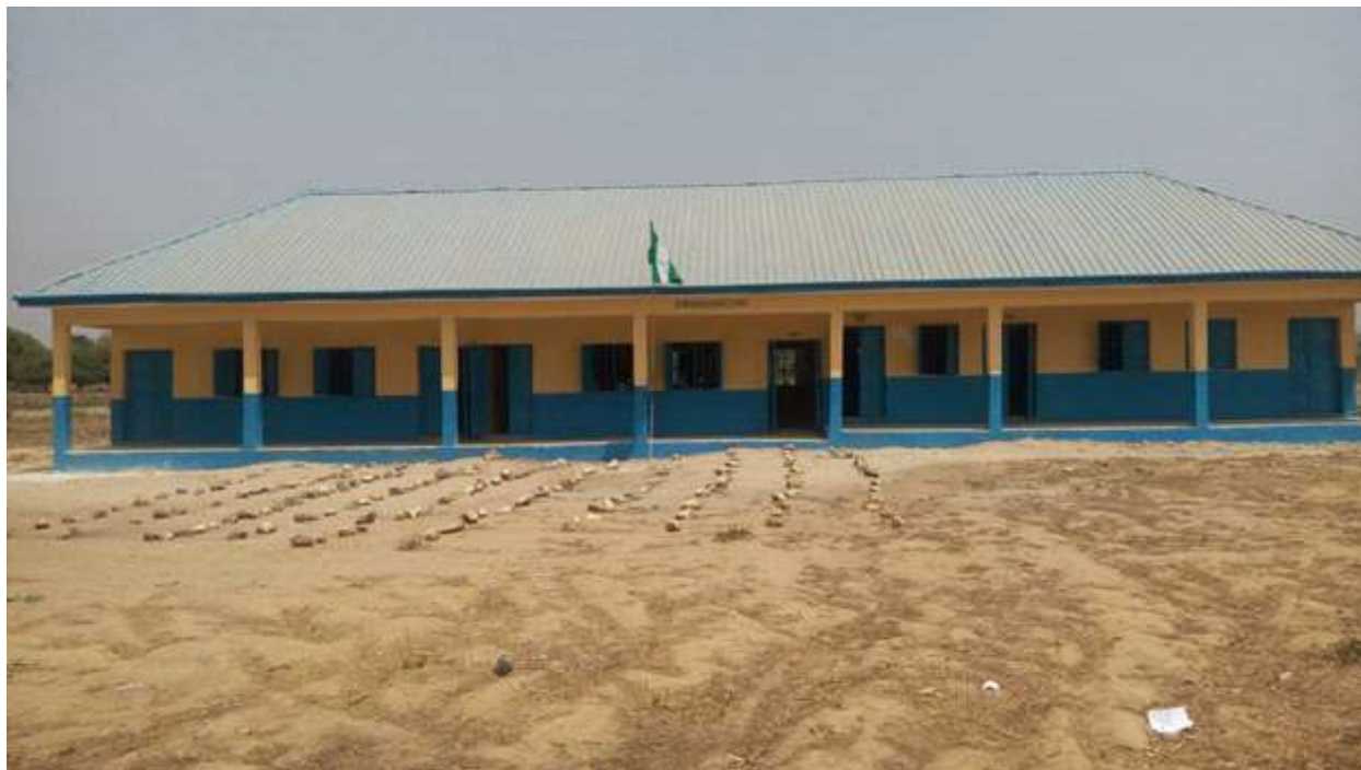
The newly constructed and furnished block of three classrooms in Kadna Community
